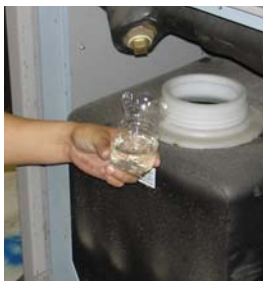
Cooling fluid levels and cleanliness can be determined with simple visual inspections. Instruments such as refractometers should be used to verify that the antifreeze properties of the cooling fluid are still adequate.
