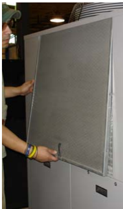
Regularly inspecting and cleaning the chiller's air filters helps ensure optimum cooling performance.
